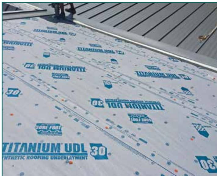
**“HIGHLY ENGINEERED, MECHANICALLY ATTACHED, COATED WOVEN SYNTHETIC ROOFING UNDERLAYMENT DESIGNED FOR SLOPED ROOFS.”**
