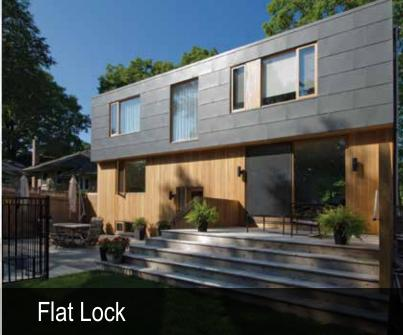
The versatility of the Flat Lock panel allows for very fast and easy installation which makes it very affordable for residential as well as commercial use. Based on a modular panel system Flat Lock delivers a more traditional rectangular design.
