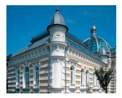
Tiles have gained popularity for roofing. Unlike sheets or shingles of similar appearance, these have forward bent edges along the lower surface to form simple interlocking joints. Diamond, Rectangular and Square-shaped tiles provide aesthetically pleasing solutions, especially for geometrically complicated building designs with roof pitches greater than 3:12.
