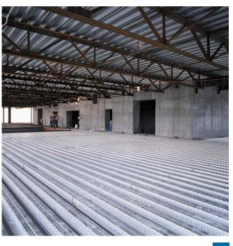
**Steel Core**: A steel deck is an engineered product and must be manufactured from sheet steel with certified structural properties. The data sheets available from the manufacturer will list the relevant material specifications and engineering properties.
