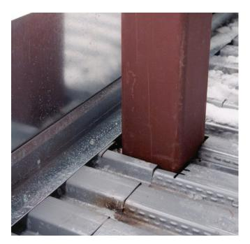
formed over supports. Side laps of adjacent units shall be mechanically fastened, or welded at intervals not greater than 900 mm. Closer spacing may be required for diaphragm action, as determined by design.
