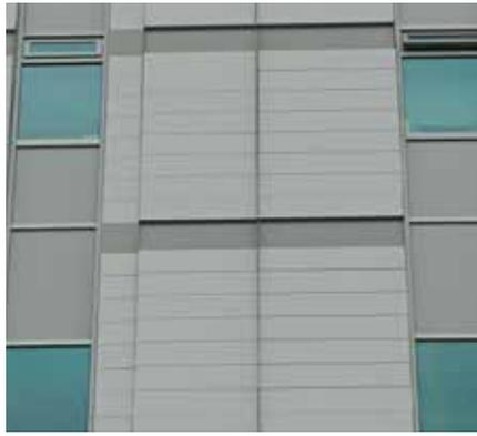
Each panel was custom designed and manufactured at the Agway Metals plant. The steel pushes in and out as it wraps around the building to “express and articulate the facade.”
