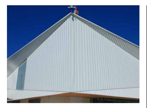
MJMA wanted each plane to be clad in white standing seam AR-25, with all of the seams perfectly aligned.
