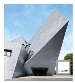
RHEINZINK is the world's leading brand of architectural-zinc for building applications. Generically known as "titanium-zinc", RHEINZINK is a natural-weathering metal that forms a grey patina after repeated exposure to moisture and air. Combining 99% special high-grade zinc with approximately 1% titanium and copper, the RHEINZINK alloy can help provide long-term solutions for roofs, facade cladding and gutters.
